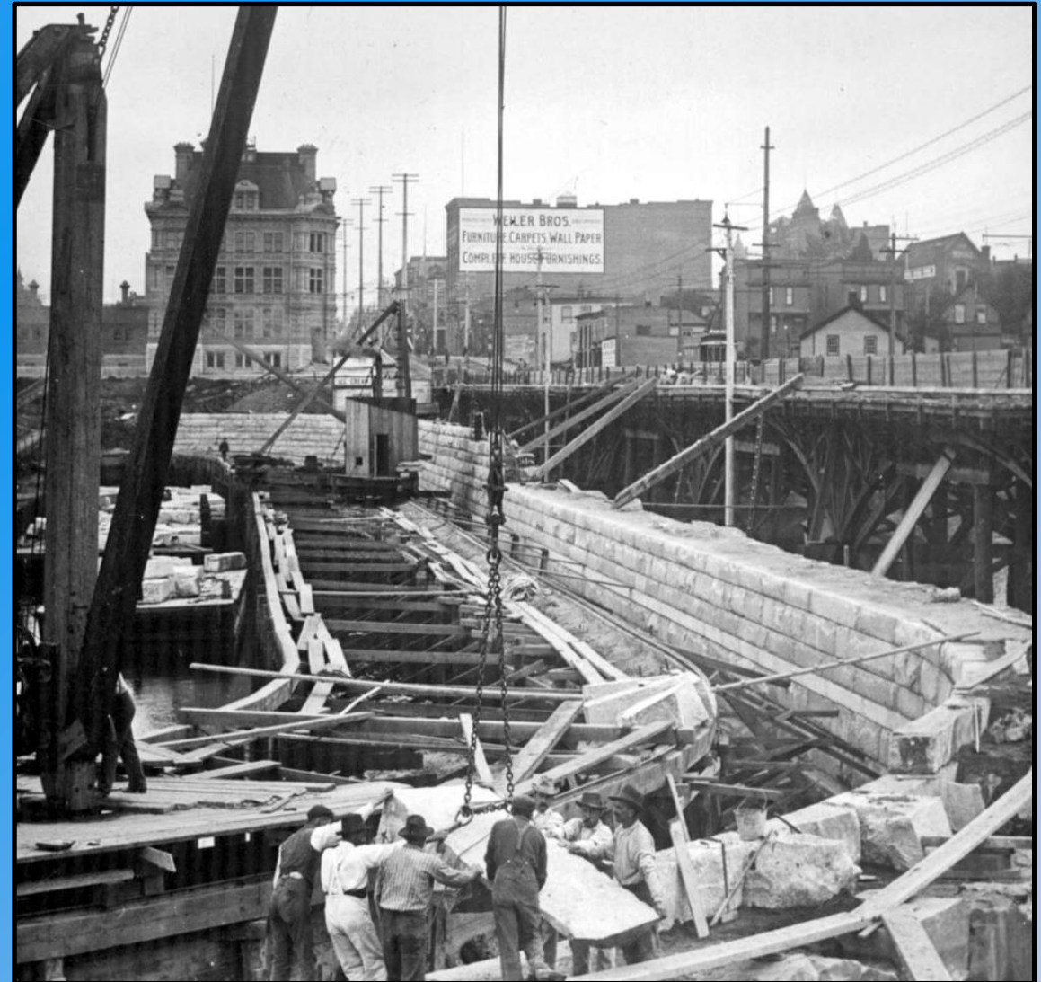
View of Inner Harbour Causeway retaining wall construction
